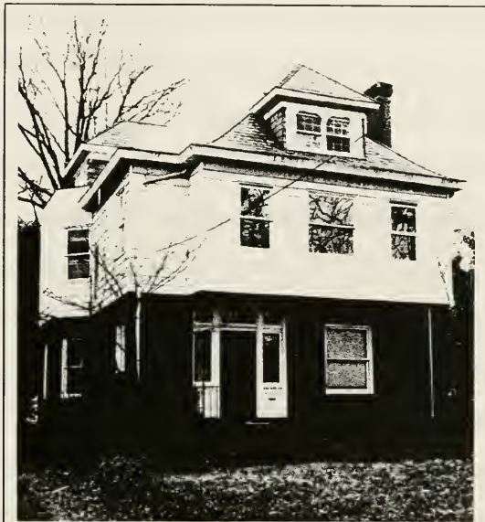
Figure 15. 908 West State Street Trenton, NJ. The building was decertified as a contributing element to the Berkley Square Historic District because of the aluminum siding. Photograph by Scott Doyle.
